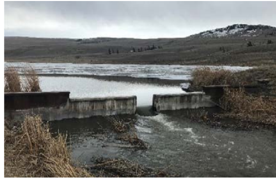
CONCRETE WEIR (VARIABLE)
